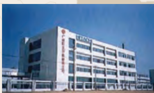
Hitachi Air Conditioning & Refrigerating, Китай
