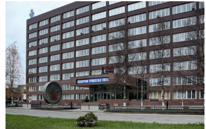
Administration building of Gazprom Transgaz Ukhta LLC Daikin VRV
