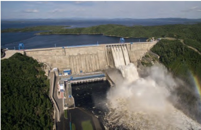
Novobureyskaya HPP, Amur region Daikin VRV
