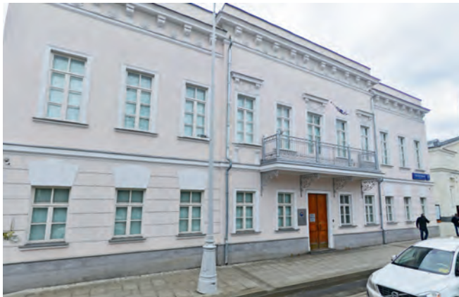
CULTURAL Centre of the Embassy of the Republic of Korea, Moscow, Chistoprudny Boulevard, 17 Hitachi mini-VRF
