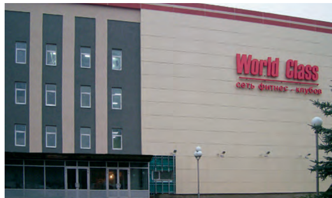
Fitness center World Class, St. Petersburg Dantherm CDP dehumidifiers
