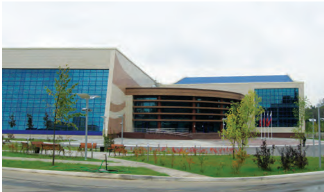
Sports centre «Ozero Krugloye», Moscow region Air supply units Dantherm DanX 12/24, decentralised ventilation system Hoval
