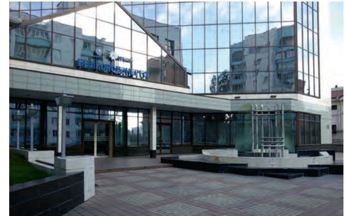
Administrative Building of the Network Control Center of IDGC of Centre – Belgorodenergo, Belgorod Hltachi VRF Set Free
