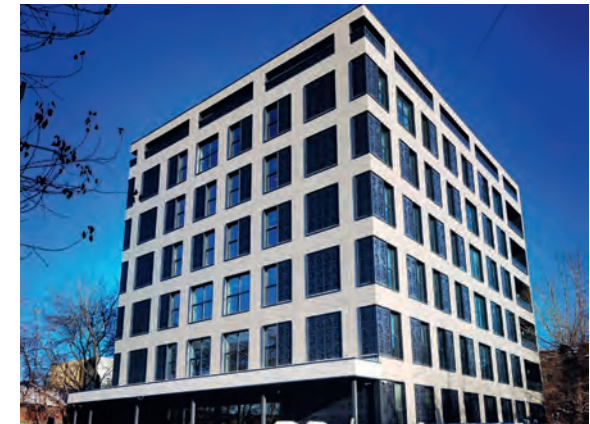
Research Institute «Heart Clinic», Yekaterinburg Multizone air conditioning system Samsung DVM S
