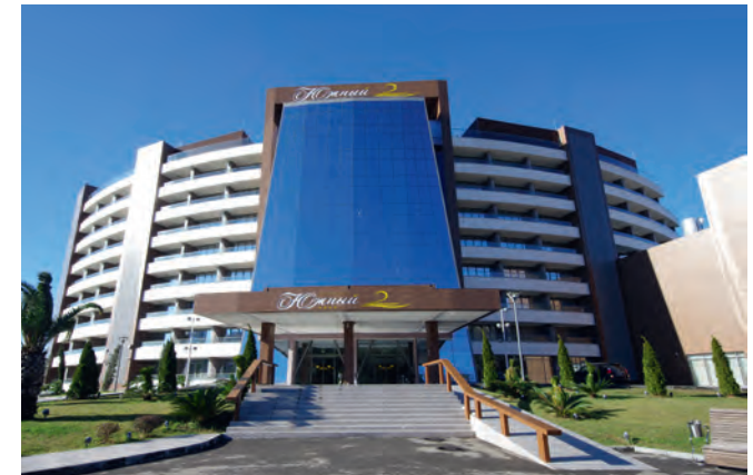
Boarding house «Yuzhnyy», Sochi Air supply units Dantherm DanX 16/32
