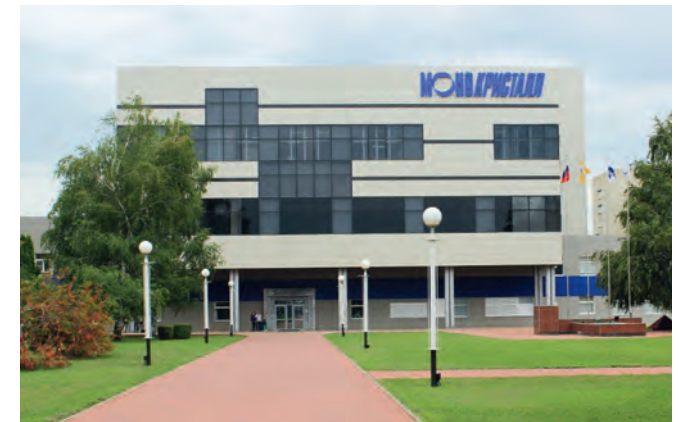
«Monocrystal» plant, Stavropol Refrion dry coolers with irrigation
