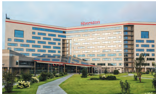
Sheraton Hotel, Moscow Daikin VRV, air supply units Dantherm DanX 7/14
