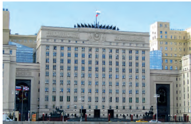
The building of the Ministry of defense of the Russian Federation on Frunzenskaya Embankment, Moscow CCU TECNAIR LV, Daikin VRV chillers
