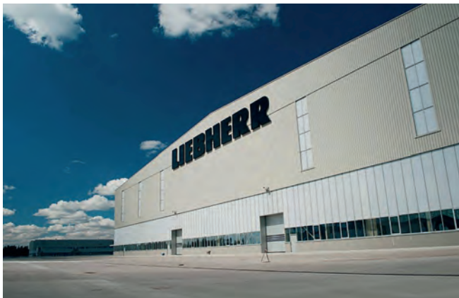
Production facilities of the Liebherr conglomerate, Dzerzhinsk, Nizhny Novgorod region Decentralised ventilation system Hoval
