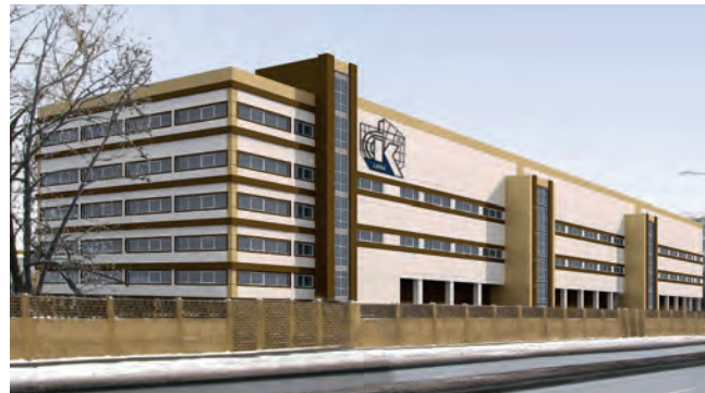
FSUE Krylov State Research Centre, St. Petersburg Decentralised ventilation system Hoval, adsorption dehumidifiers Cotes
