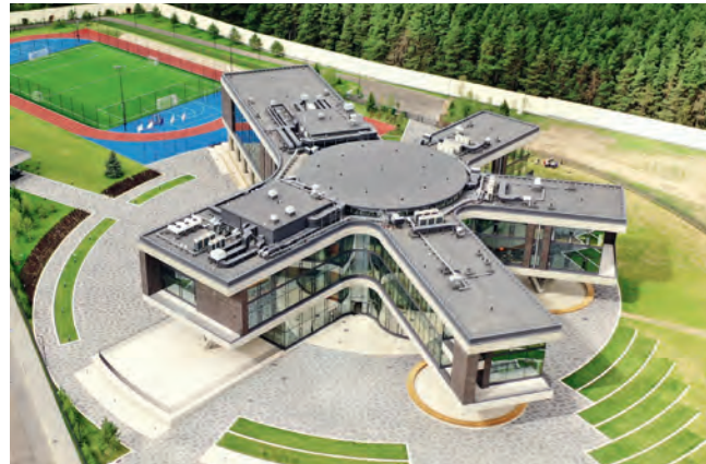
Wunderpark International School, Moscow region Decentralised ventilation system Hoval
