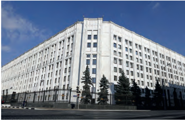
The building of the Ministry of defence of the Russian Federation, Moscow Daikin VRV chillers
