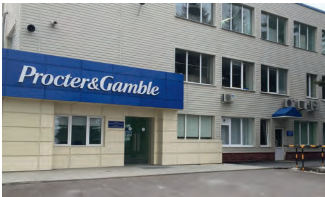
Procter & Gamble manufacturing facilities, Moscow region Decentralised ventilation system Hoval
