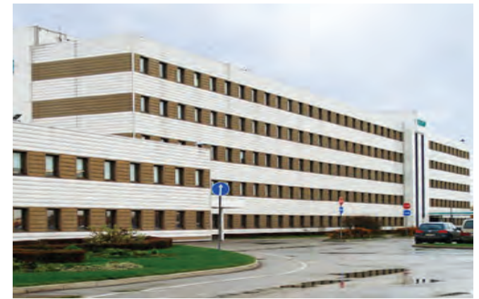
Warehouse complex «Petro», St. Petersburg Decentralised ventilation system Hoval
