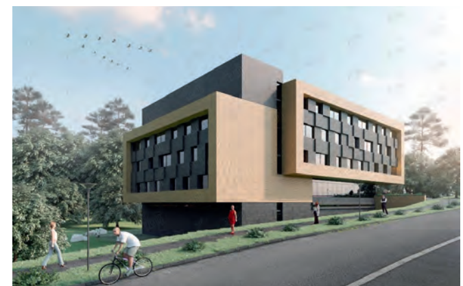
Multipurpose medical centre, Vladivostok Multizone air conditioning system Samsung DVM S
