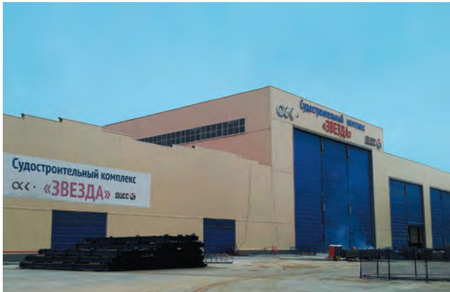
Shipbuilding facility «ZVEZDA», Vladivostok Decentralised ventilation system Hoval, adsorption dehumidifiers Cotes
