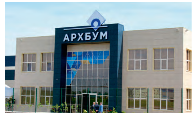
Production and distribution facilities of the Arkhbum company, Kaluga region and Moscow region Decentralised ventilation system Hoval
