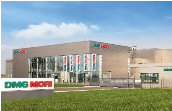
Ulyanovsk Machine Tool Factory DMG Mori, Ulyanovsk Decentralised ventilation system Hoval
