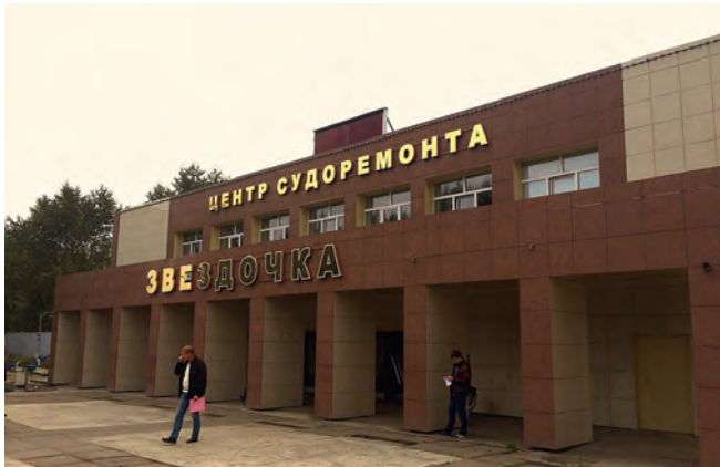
Ship-repairing centre «Zvyozdochka», Severodvinsk Decentralised ventilation system Hoval
