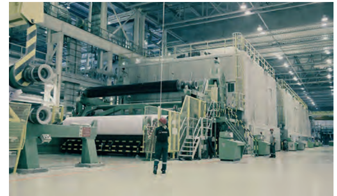
Bratsk timber processing complex (ILIM Pulp Enterprise), Bratsk CCU TECNAIR LV
