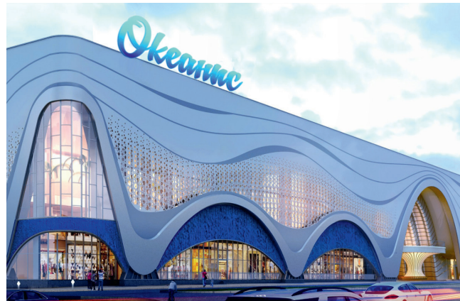
Multifunctional complex «OCEANIS», Nizhny Novgorod Daikin VRV chillers, air supply units Dantherm DanX 16/32
