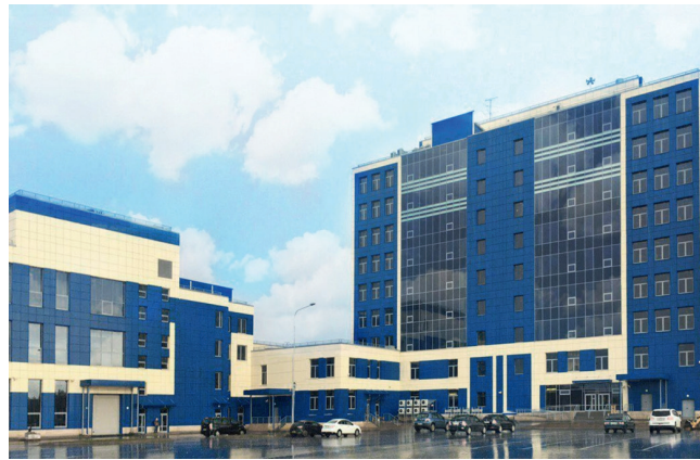
«Pharmasyntez-Nord» warehouse facilities, St. Petersburg Decentralised ventilation system Hoval
