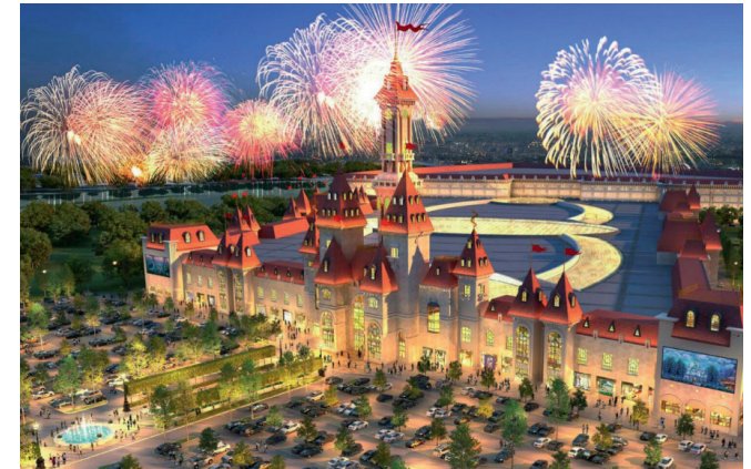
Amusement park «Dream Island», Moscow Decentralised ventilation system Hoval
