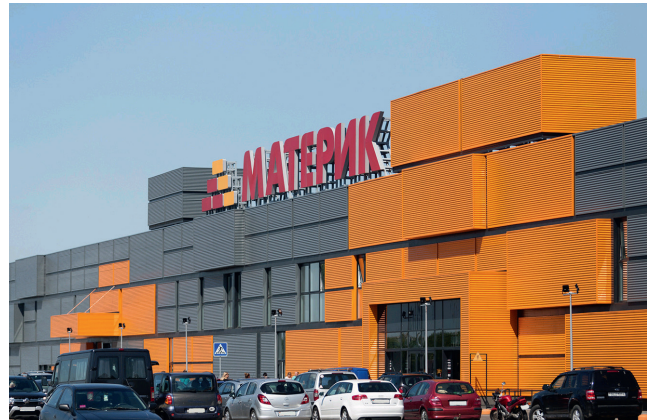
Hypermarket of construction materials «Materik», Republic of Belarus Decentralised ventilation system Hoval
