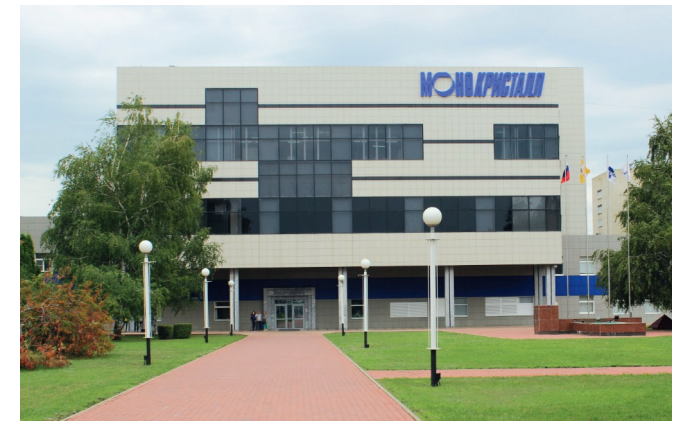
«Monocrystal» plant, Stavropol Refrion dry coolers with irrigation
