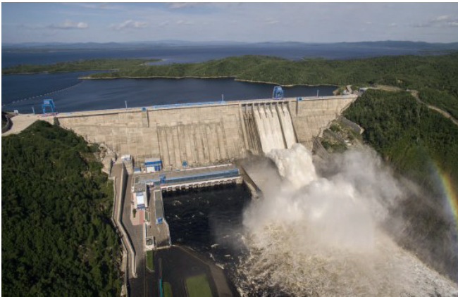
Novobureyskaya HPP, Amur region Daikin VRV
