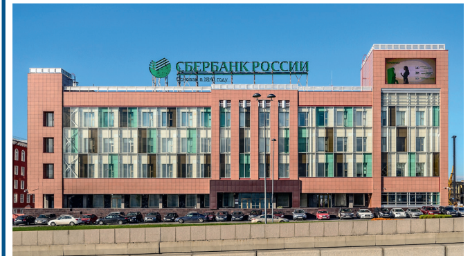
Administration building of JSC «Sberbank of Russia», St. Petersburg Daikin VRV
