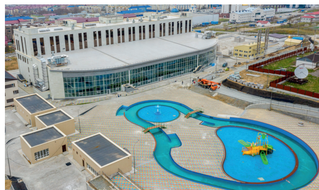
Water park, Yuzhno-Sakhalinsk Air supply units Dantherm DanX 9/18 XKS
