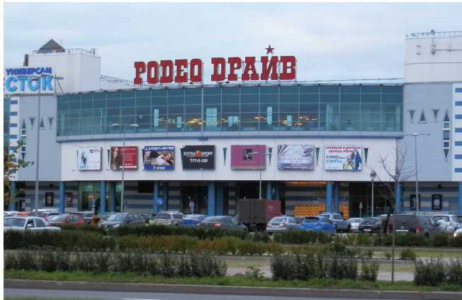
Water park «Rodeo Drive», St. Petersburg Air supply units Dantherm DanX, decentralised ventilation system Hoval
