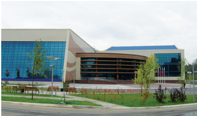
Sports centre «Ozero Krugloye», Moscow region Air supply units Dantherm DanX 12/24, decentralised ventilation system Hoval
