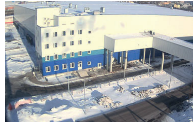
Customs and warehouse facility «Transservice», Moscow region, Pushkinsky district, Tarasovka Daikin VRV
