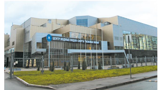
Water Sports Center «Nevskaya Volna», St. Petersburg Air supply units Dantherm DanX 12/24
