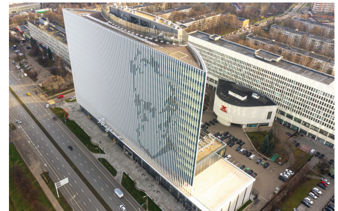
Rostelecom office, business center «Akademik», Moscow Hltachi VRF Set Free
