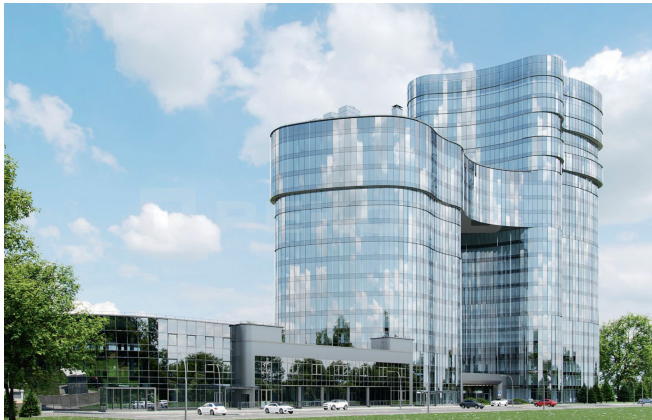
Business Centre «Sea Capital», St. Petersburg Absorption chiller York, total power capacity 3 mW
