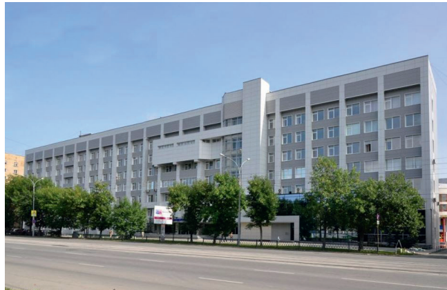
Office building «Uralzheldorproekt», Yekaterinburg Hitachi VRF Set Free
