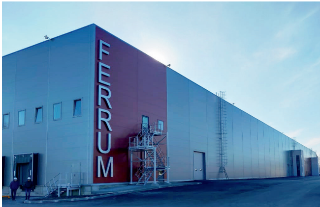
Ferrum steel production plant, Voronezh Decentralised ventilation system Hoval
