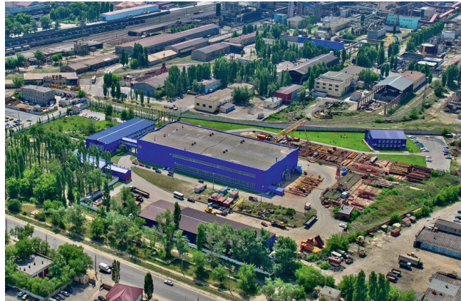
Novolipetsk Iron & Steel Works, Lipetsk Hitachi VRF Set Free
