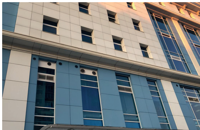
«Cargill» Company premises, Krasnodar Hitachi VRF Set Free
