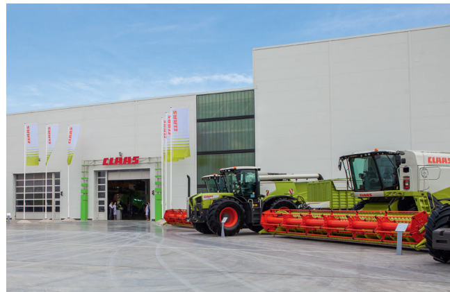
CLAAS production facilities, Krasnodar Decentralised ventilation system Hoval
