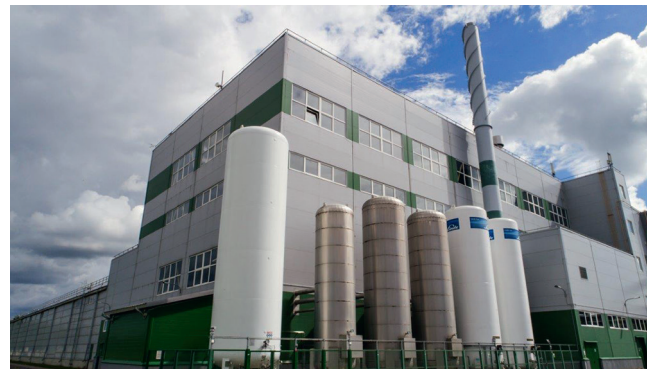
«JTI Kres Neva», non-tobacco components production building, Leningrad region AHU York, total air flow 81,000 m³/h, Daikin VRV chillers
