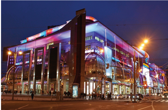
Shopping and Entertainment Center "Evropeisky, Moscow Construction and installation works of Daikin VRV systems. Reconstruction of the 7th and 8th floors of the building
