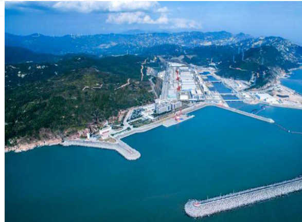
Yangjiang nuclear power plant , Guangdong, China
