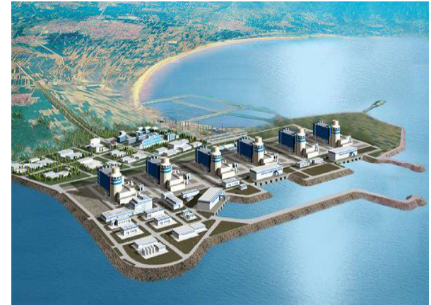
Haiyang nuclear power plant, Shandong, China
