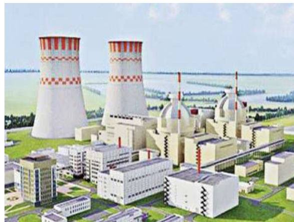
Rooppur nuclear power plant, Bangladesh
